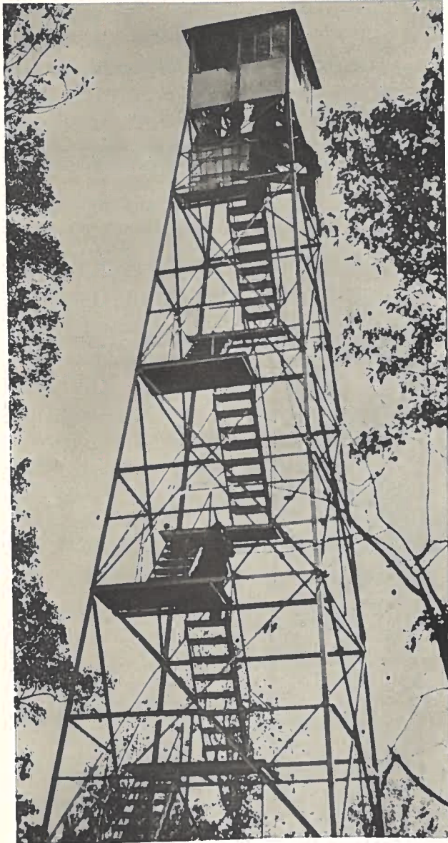
Tower completed in 1953.
